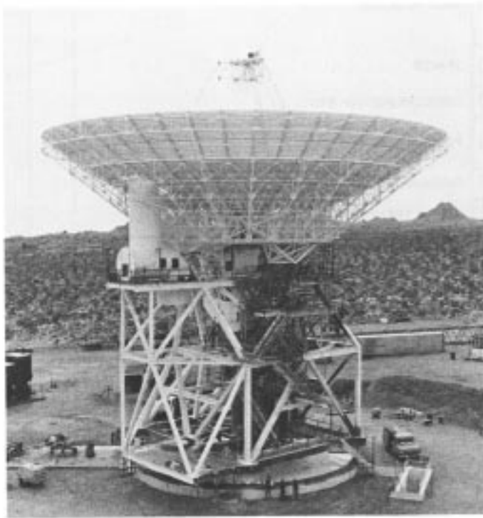
Fig. 1. The 34-m BWG antenna nearing completion of the construction phase.
