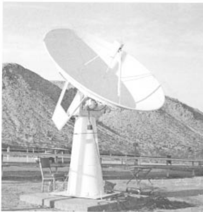
Fig. 2. Newly installed 10-ft reference antenna.
