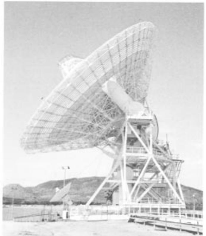
Fig. 3. View of the 34-m antenna and the 10-ft reference antenna pointed at a geostationary satellite at a 46.5-deg elevation angle.
