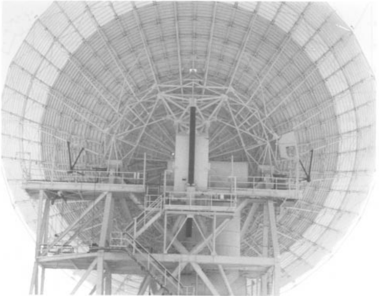
Fig. 5. X-actuators in place.
