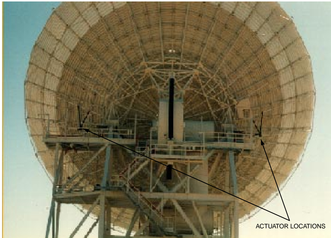
Fig. 1. Cammatic actuator locations.
