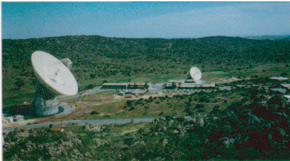
Fig. 2. DSN antennas at Robledo and the surrounding hills: the 70-m antenna on the left and the ridges in the background at a higher elevation, blocking the view toward Madrid.
