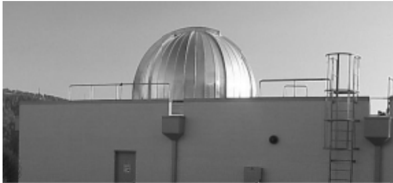
Fig. 1. JPL's Optical Communications Telescope Laboratory is located on Table Mountain in Wrightwood, California. The laboratory stands at a 2.2-km altitude and will house a 1-m telescope.
