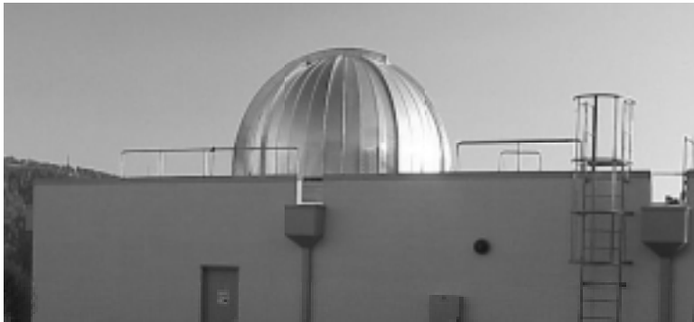
Fig. 1. The OCTL telescope building and dome at Table Mountain Facility in Wrightwood, California.
