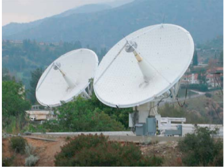
Fig. 3. Antennas at JPL: (a) 12-m-diameter antenna and (b) 6-m-diameter antennas.
