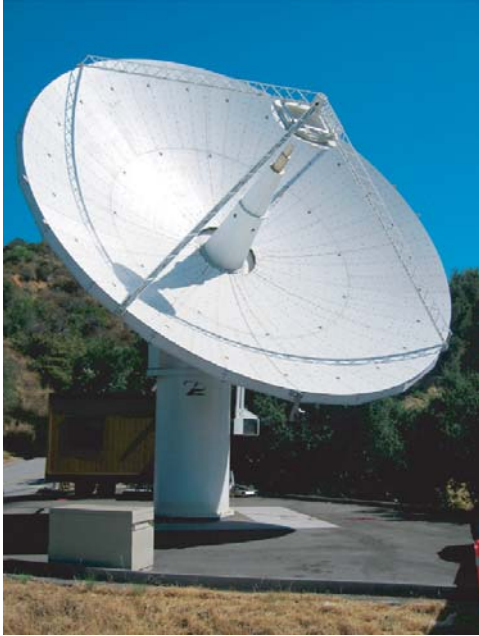
Fig. 3. Antennas at JPL: (a) 12-m-diameter antenna and (b) 6-m-diameter antennas.
