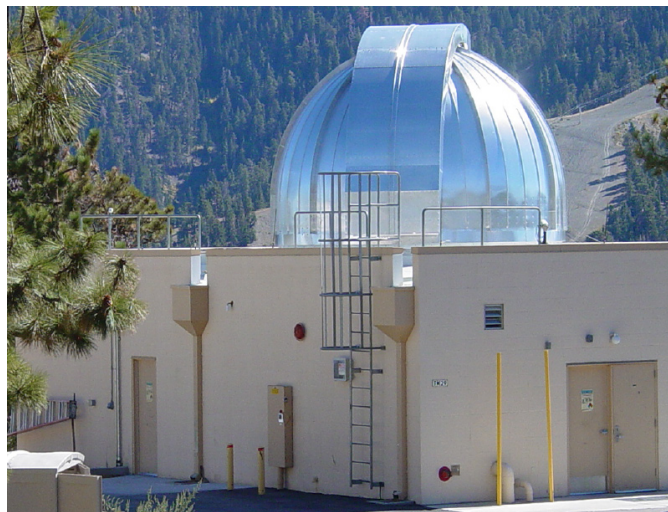
Figure 1. The OCTL facility at Table Mountain houses a 1-m azimuth/elevation coudé focus telescope.
