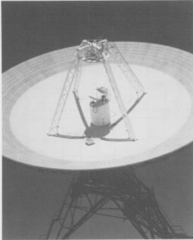
Fig. 1. DSS 12 34-m HA-Dec antenna with S/X reflex feed system
