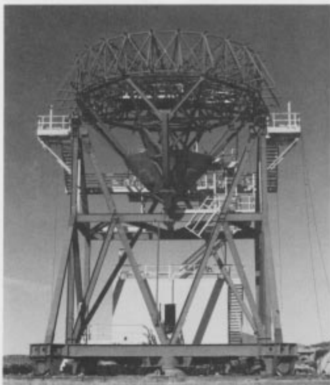
Fig. 9. Main reflector support structure, DSS 15
