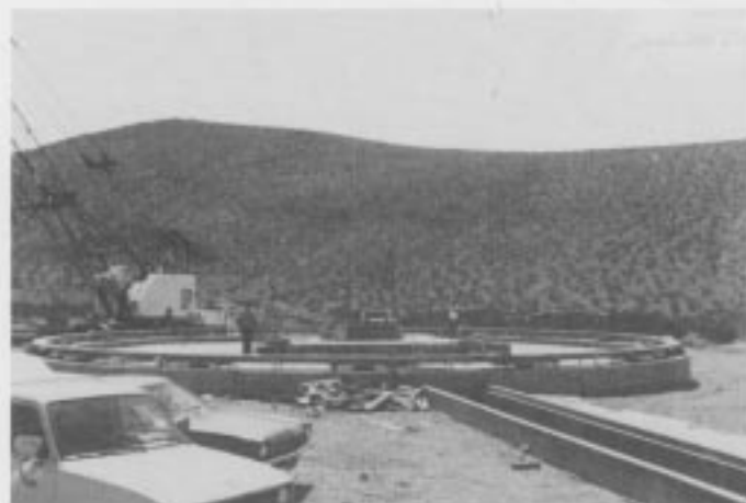
Fig. 6. Track and support runner, DSS 15
