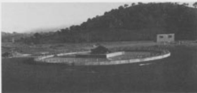
Fig. 2. Foundation, 34-m Az—EI antenna, DSS 45
