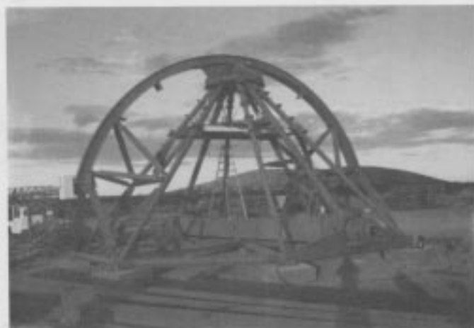
Fig. 8. Tipping structure support and elevation bearing
