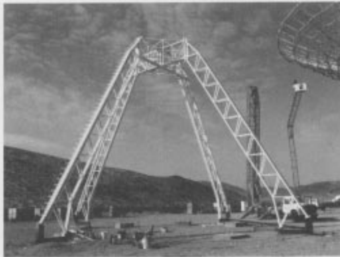
Fig. 13. Quadripod structure, DSS 15
