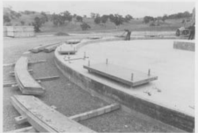
Fig. 3. Track foundation and runner support
